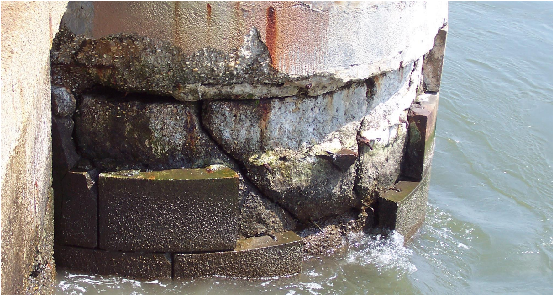
Tower Damage
