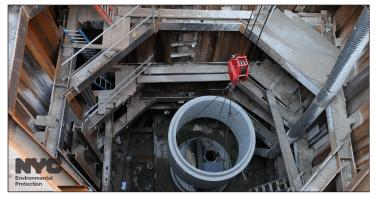
Work to repair the compromised sewer line on 92<sup>nd</sup> Street in Bay Ridge continues to progress and during the last week concrete sections of manhole were set in place and the hole has been back-filled from a depth of approximately 70 feet to 17 feet. Work to repair the local sewer line is now underway and the final sections of manhole have been delivered. BWSO has made remarkable progress on the complex repair of this sewer line.
