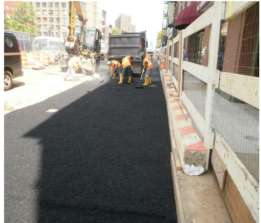
Temporary Pavement Restoration
