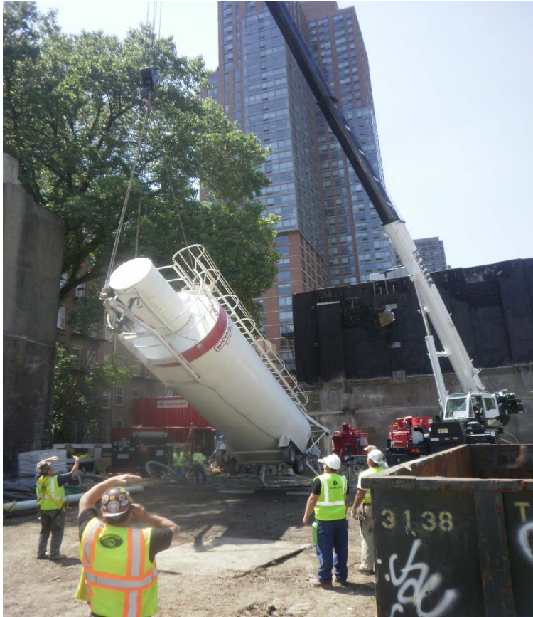
Grouting Silo Installation – Ancillary No. 2
