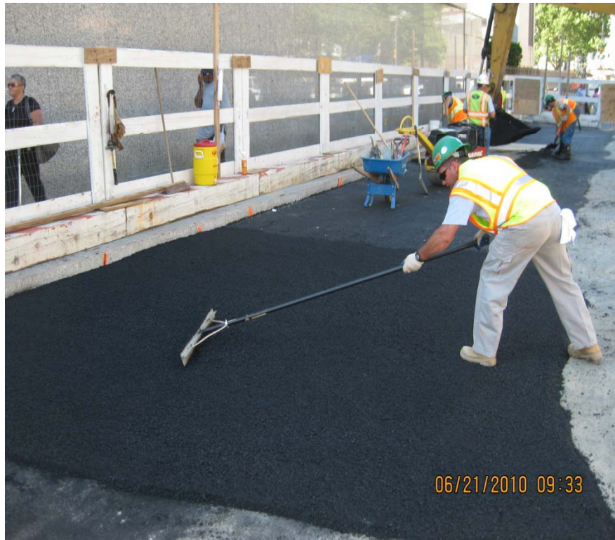
Temporary Pavement Restoration
