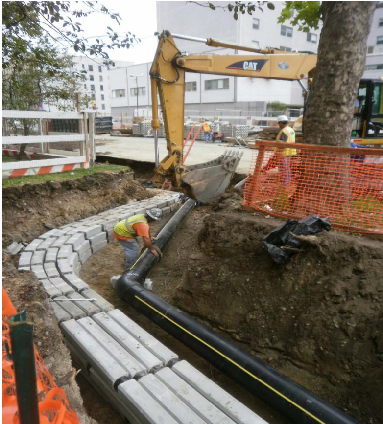
Installation of Conduits & Gas Main
