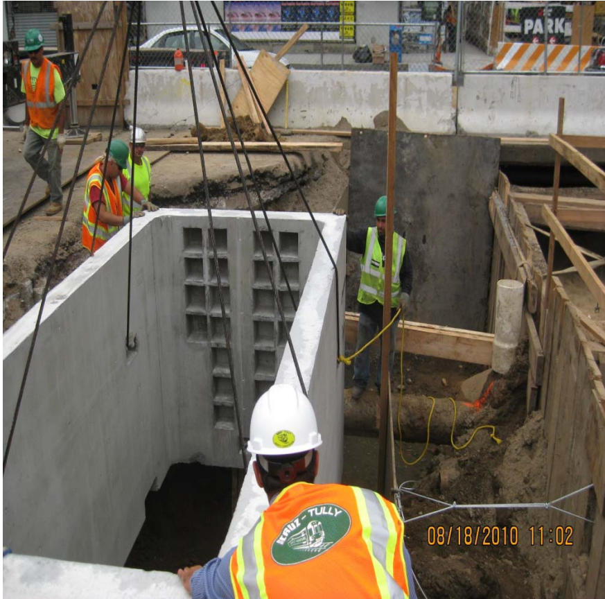
Electrical Manhole Installation – 2 nd Avenue at 96 th Street
