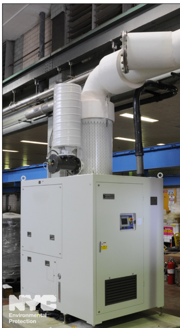
A new low-horsepower, high-speed blower for low demand periods has been installed at the Rockaway Wastewater Treatment Plant. If the trial period is successful, ACE funds will be used to purchase the blower for permanent use. A similar blower will replace an existing high-horsepower blower at the Bowers Bay Wastewater Treatment Plant.
