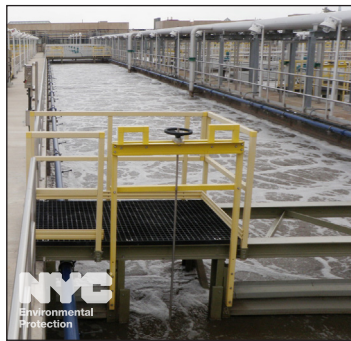
High-efficiency fine bubble ceramic diffusers will be installed in the aeration tanks of the Coney Island Wastewater Treatment Plant. The current diffusers have been in operation for over 17 years and are nearing the end of their useful life.
