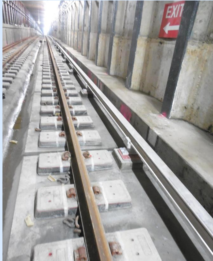
LVT Track installed with Aluminum 3 rd rail
