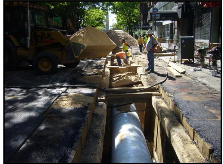
Workers perform backfilling of the 36" trunk water main trench on E. 59<sup>th</sup> St. between 2<sup>nd</sup> Ave. and 3<sup>rd</sup> Ave.
