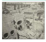
Photo from June 18, 1912 showing the lower gate chamber of the Catskill Aqueduct Headworks, which were a labyrinth of subsurface tunnels and chambers equipped with valves, sluice gates, and operating equipment. They release water from the Ashokan Reservoir into the Catskill Aqueduct and can route millions of gallons of water each day. The lower gate chamber is on the downstream side of the
