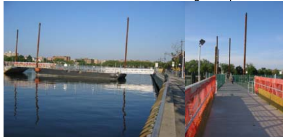
2005: Pontoon Bridge Used During the Emergency Reconstruction of the Ocean Avenue Pedestrian Bridge over Sheepshead Bay. (Credit: Russell Holcomb)
