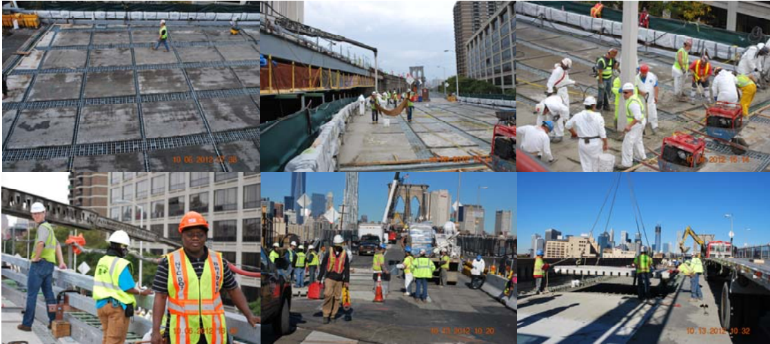
First Full Roadway Closure: Manhattan Approach, Ramp A Concrete Placement. Engineer-in-Charge Ohene Duodu at the Site. Second Full Roadway Closure: Brooklyn Approach, Brooklyn Bound Roadway Super Slab installation - Installing Super Slab.
