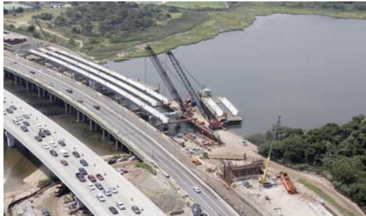
Paerdegat Basin- Eastbound Belt Parkway Traffic on New Eastbound Bridge Shown at Left. Westbound Belt Parkway Traffic on Old Paerdegat Basin Bridge at Center. Tub Girder Erection in Progress at Right Side by Crane on a Temporary Work Platform at Future Westbound Bridge.
