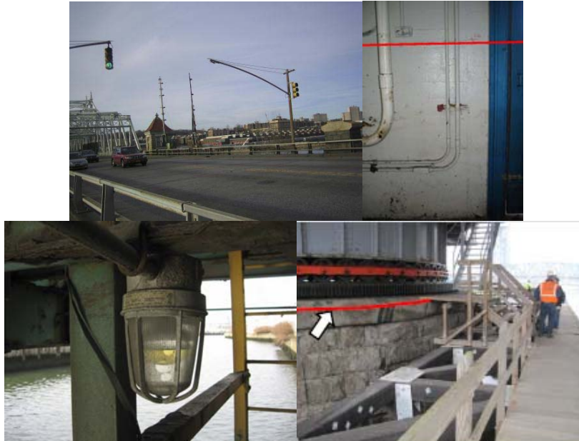
East End of the West 207 th Street Bridge - Missing Traffic Signal was Knocked Down by the Hurricane Winds. Borden Avenue Bridge Operator's House Basement Level – Depicted Flood Line was Approximately 5 Feet Above the Floor. Grand Street Bridge – Standing Water in the Access Light Fixture at the East Wedge Walkway. Madison Avenue Bridge - General View of Fender and Center Pier—the Red Line Depicts the Approximate Water Level.
