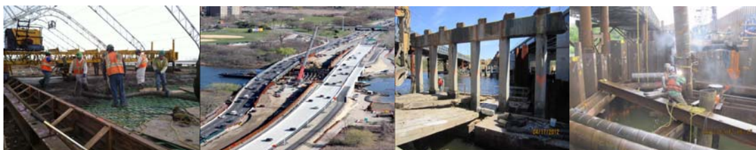
Fresh Creek Bridge in February 2012: Concrete Placement. Fresh Creek Bridge in April 2012: Facing East. New Eastbound Approach Roadways, Bridge Deck, Bicycle/Pedestrian Walkway on Right. Temporary Bridge for Westbound Traffic at Left. Old Bridge Demolition at Center. Fresh Creek Facing East. Stage 3 Demolition of Piers of Old Fresh Creek Westbound Bridge. Workers Cutting off Excess Steel Pipe Casing for Cast-in-Place Concrete Piles at Future Westbound Bridge. Temporary Bridge at Left.
