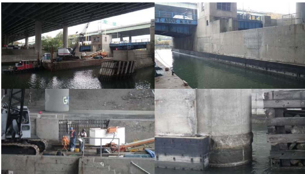
Unionport Bridge – Rebuilt the West Wall Fender System to Stop Barges From Hitting the Side of the Bridge. Safety Flags on the Concrete East Parapet Wall Were Also Completed. (Credit: Thomas Leung)
