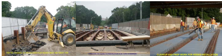
June 2012: Removing Soldier Piles Behind the West Abutment. June 2012: Formwork for Stage 2 Superstructure Slab. July 2012: Formwork for Stage 2 Deck.
