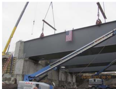
Setting the Last Tub Girder Section for the Westbound Bridge at the East Abutment.
