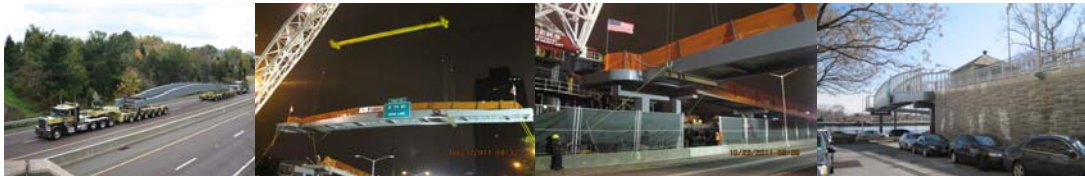
The New Bridge Span in Transit from Just North of Philadelphia to Jersey City. It was Then Loaded on the Barge and Brought up the East River to the Site. The Span Size was 26' x 135' and Weighed Approximately 80 Tons. New Main Span Steel Erection in October 2011. New West Ramp Masonry Wall.
