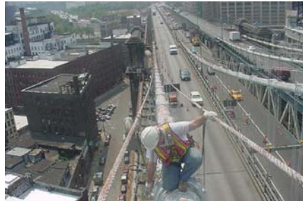
Inspector on Manhattan Bridge Cable. (Credit: NYSDOT)
