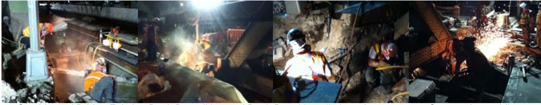
Southbound Bridge Existing Deck Demolition and Deck Panel Installation. August 2011: Stage 2 Assembling and Welding Steel Packs for Southbound Bridge.
