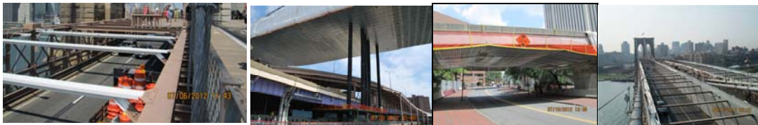
July 2012: Painting Brooklyn-Bound Top Struts. Manhattan Side Span Blasting in Progress. Platform Installation at Ramp E. August 2012: Manhattan Main Span Vertical Wall.
