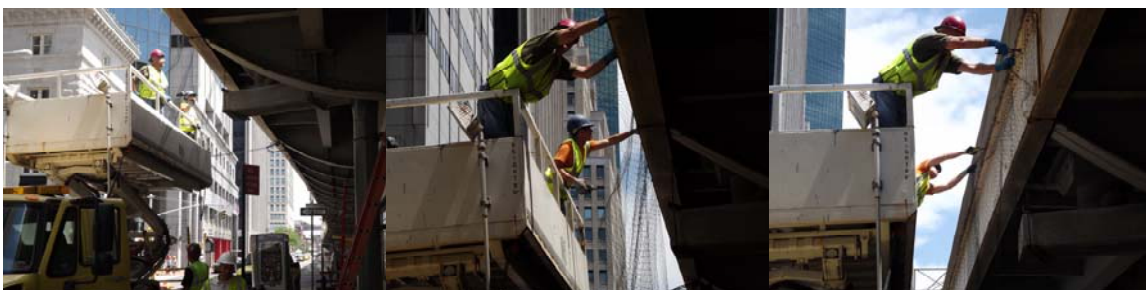
Installing Pigeon Netting at Old Slip (FDR Drive at the South Street Viaduct) in June 2012: Carpenters Stephen Buckley, William Sic, and Joseph Moschella, and Supervisor Carpenter Joseph Vaccaro. (Credit: Thomas Whitehouse)
