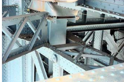
Truss Bearing on Manhattan Bridge. (Credit: NYSDOT)
