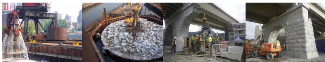
June 2011 River Work: Picking Up Waste With a Clamshell Bucket. July 2011: Demolition of Old Pier 9. March 2011: Stage III Caisson Concrete Placement at Caisson #2 at Pier 11. Setting Granite Stone Facing at Pier 11. Finished Stage VB Removal of Steel Girder at South Bay at Existing Span 15.
