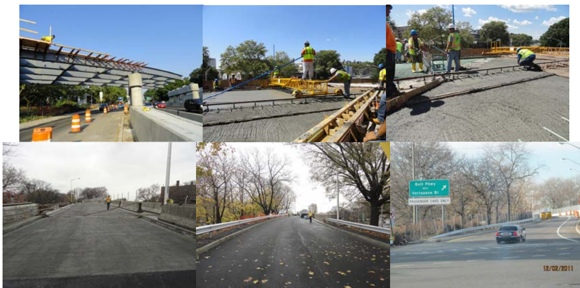
2011: Installation of Steel Girders over the South Service Road and Eastbound Belt Parkway. August 2011: Concrete Deck Placement. November 2011: Completed North and South Approach Roadways. December 2, 2011: Bridge Open to Traffic.
