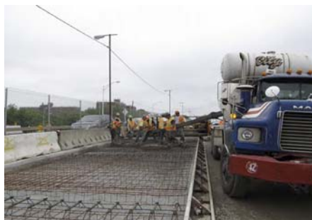
Placing and Finishing On-Grade Concrete Pavement for Westbound Roadway on West Side of the Rockaway Parkway Bridge.
