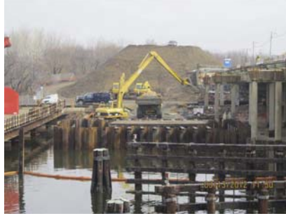
Paerdegat Basin Waterway with Partially Demolished Bridge, Temporary Work Platform, and Pier 2 Cofferdam. Embankment for Future Westbound Bridge in Background.
