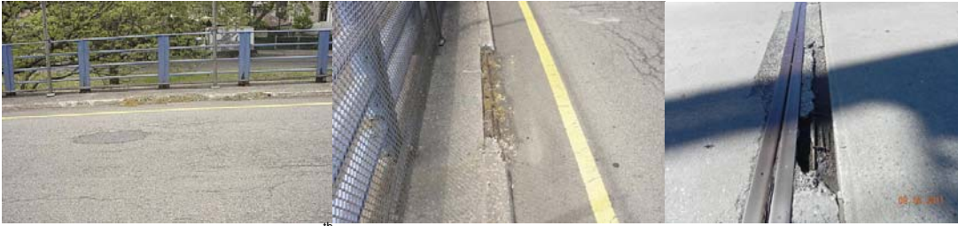
Spalled Section of Curb on the East 8 th Street Bridge in 2006. (Credit: NYSDOT) Spalling With Exposed Rebar on the Beginning Abutment Joint Header of the Westchester Avenue Bridge over the Bronx River in 2011.
