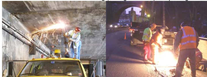
PIA Flag (Truck Wedged Under the FDR Drive at Span 41): Removing the Debris. (Credit: Victor Sandoval) PIA Flag Repair (Through Hole) on Harlem River Drive Ramp. (Credit: Bojidar Yanev)
