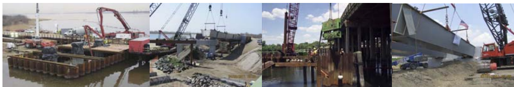
February 2011: Pumping Concrete at Paerdegat Basin Cofferdam for Pier No.3. April 2011: Setting Tub Girder Sections at Eastbound Bridge Between West Abutment and Pier No. 1. June 2011: Hammer Being Positioned to Drive Steel Sheet Piling for Cofferdam at Westbound Bridge – Pier # 2. July 2011: Setting Final Tub Girder Section at East Abutment.
