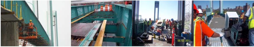
January 2011: Under-Deck Shield Installation for Manhattan Approach Span 6. April 2011: Removing Concrete Decking Material. June 2011: Pouring Concrete Decking at Span 7.
