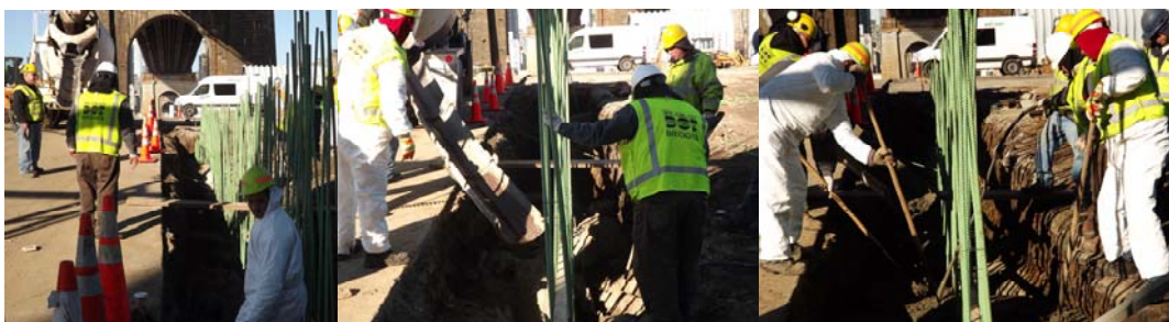
December 2012: Preparing a Footing for a Concrete Pad That Will Hold Office Trailers and Storage Containers in the Vernon Boulevard Yard Under the Ed Koch - Queensboro Bridge. (Credit: Thomas Whitehouse)
