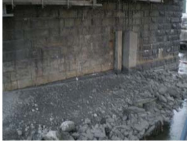
Eroded Riprap Pier Protection at Pier 11 of Old Willis Avenue Bridge in 2008. (Credit: NYSDOT)
