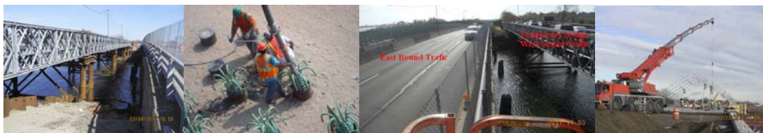
Fresh Creek Bridge March 2011: Westbound Temporary Bridge at Left, Existing Bridge at Right. July 2011: Concrete Pouring in Piles. November 2011: The Remaining Bridge Carrying East Bound Traffic and Temporary Bridge Carrying West Bound Traffic. (Credit: NYSDOT) December 2011: Commenced Installation of Winter Tent Enclosure for Stage IIB Concrete Bridge Deck Placement. (Tent Credit: Daniel Horn)
