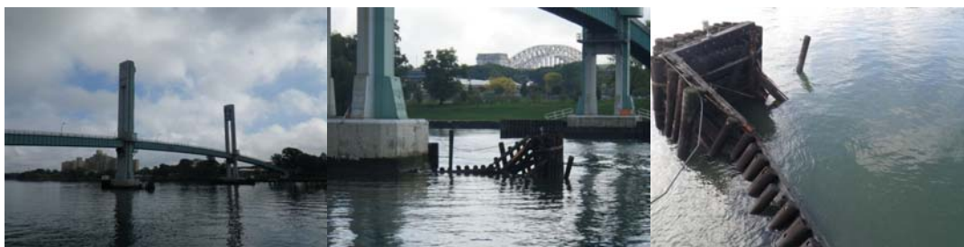
Emergency Inspection on Wards Island Bridge Revealed that the Southwest Fender System Collapsed and Required Repairs.
