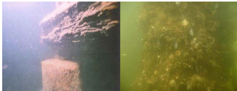
Severe Marine Borer Infestation in Timber Cribbing of Carroll Street Bridge and Moderate Marine Growth Below Waterline on the Ocean Avenue Pedestrian Bridge in 2009. (Credit: NYSDOT)
