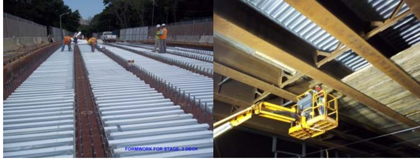
July 2012: Formwork for Stage 2 Deck. December 2012: Removing Shielding and Formwork.
