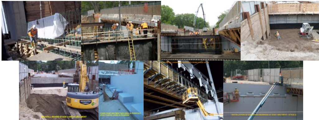
Shore Road Circle Bridge in April 2012: Placing Concrete for Stage 2 West Abutment Footing. May 2012: Stage 2 Backfill Behind East Abutment. East Abutment Backwall Rebar Installation. June 2012: Backfill Behind Stage 2 West Abutment. Painting of East Abutment Back Wall and Pedestals. June 2012: Removing Brackets from Stage 1A/1B. Installing Expansion Bearings at East Abutment in Stage 2.
