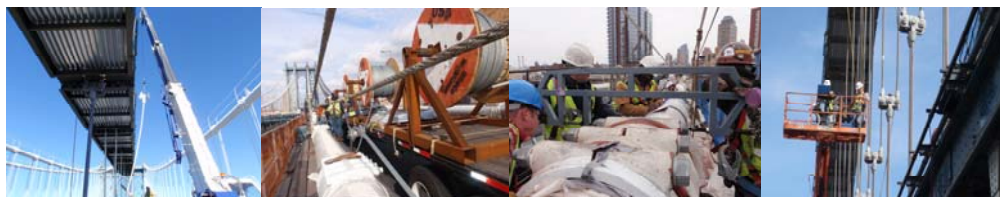
March 2011: Removal of Existing Suspender, 'C' Truss. April 2011: Installation of New Hand Ropes for 'C' Cable. April 2011: Checking Bolt Tension in New Cable Band Bolts. August 2011: Checking Suspender Loads With an Accelerometer.
