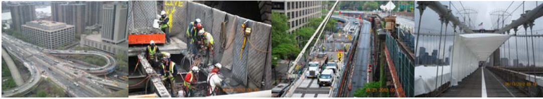
April 2012: Overview. (Credit: Maria Mikolajczyk) Manhattan Approach, Ramp A Existing Deck Demolition. June 2012: Brooklyn Side Span Netting Protection for Main Cable and Suspender Rope Painting.
