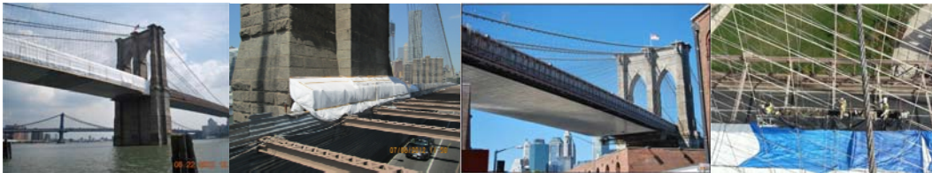
August 2012: Manhattan Side Span Containment at Manhattan Tower. Brooklyn Side Span Protective Shield. Brooklyn Side Span Suspender Ropes Painting.
