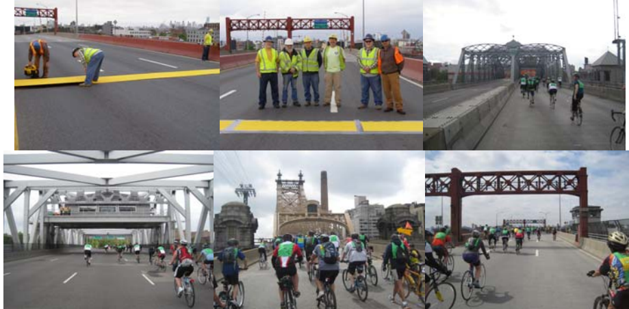
Preparing the Pulaski Bridge for the Bike Tour by Installing Plywood Covers Over the Finger Joints. Blowing Out Debris, Placing the Plywood Board, and Taping into Place: Carpenters Mark Pavia, Michael Short III, and Patrick Burns. Completed Job: Carpenter Patrick Burns, Supervisor Carpenter John Motylewski, and Carpenters John Green, Andrew Myjer, Michael Short III, and Mark Pavia. (Credit: Paul Schwartz) Cyclists on the Madison Avenue, Third Avenue, Ed Koch Queensboro, and Pulaski Bridges. (Credit: Mark Feinman)
