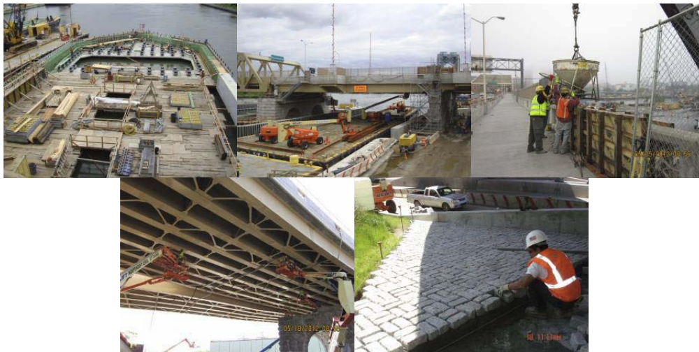
May 2012: Pier 6 North Fender. Touch-up Paint Operations at the Underside of Span 5. Finished Span 10 Parapet Wall Concrete Placement. Girder Touch-up Painting at Span 12. Preparing and Installing Granite Stone Pavers at Ramp-C End Abutment.
