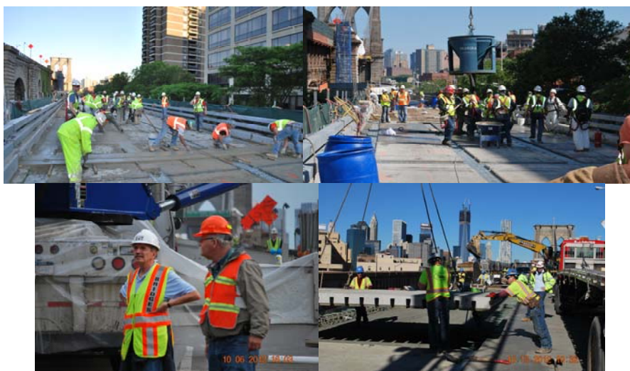
First Full Roadway Closure in October 2012: Manhattan Approach, Ramp A Concrete Placement. Chief Bridge Officer Henry D. Perahia and Deputy Chief Engineer Robert Collyer at the Site. Second Full Roadway Closure: Brooklyn Approach, Brooklyn Bound Roadway Super Slab installation - Installing Super Slab.
