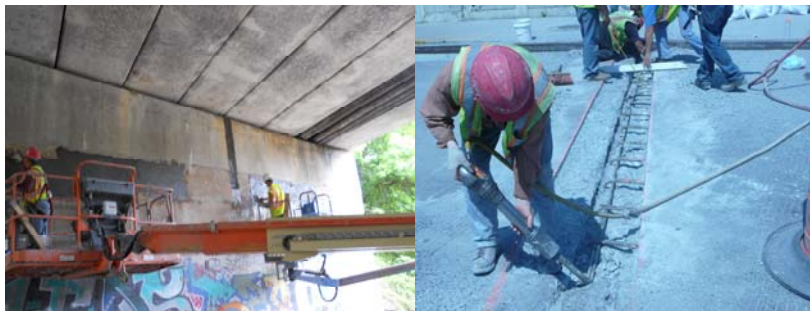
15 th Avenue Bridge - Vertical Patch Repair on the Abutment Wall. Joint Repair Work.
