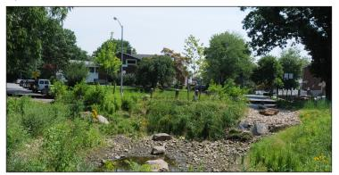
EP's award-winning Bluebelts are expanding in Queens. Based on the term "greenbelt," used to describe a large area of parkland in Staten Island, DEP's "Bluebelts" provide ecologically sound and cost-effective stormwater management. Through preservation of natural drainage corridors, such as streams, ponds, lakes,
