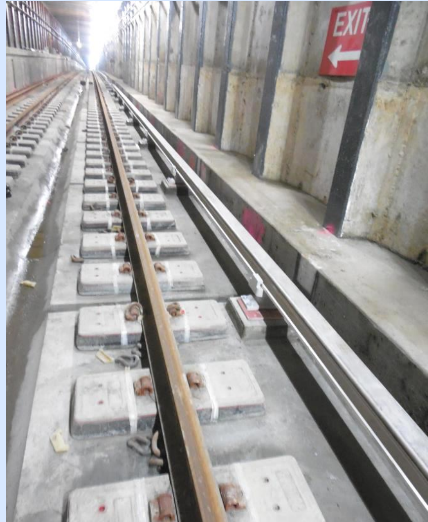
LVT Track installed with Aluminum 3 rd rail
