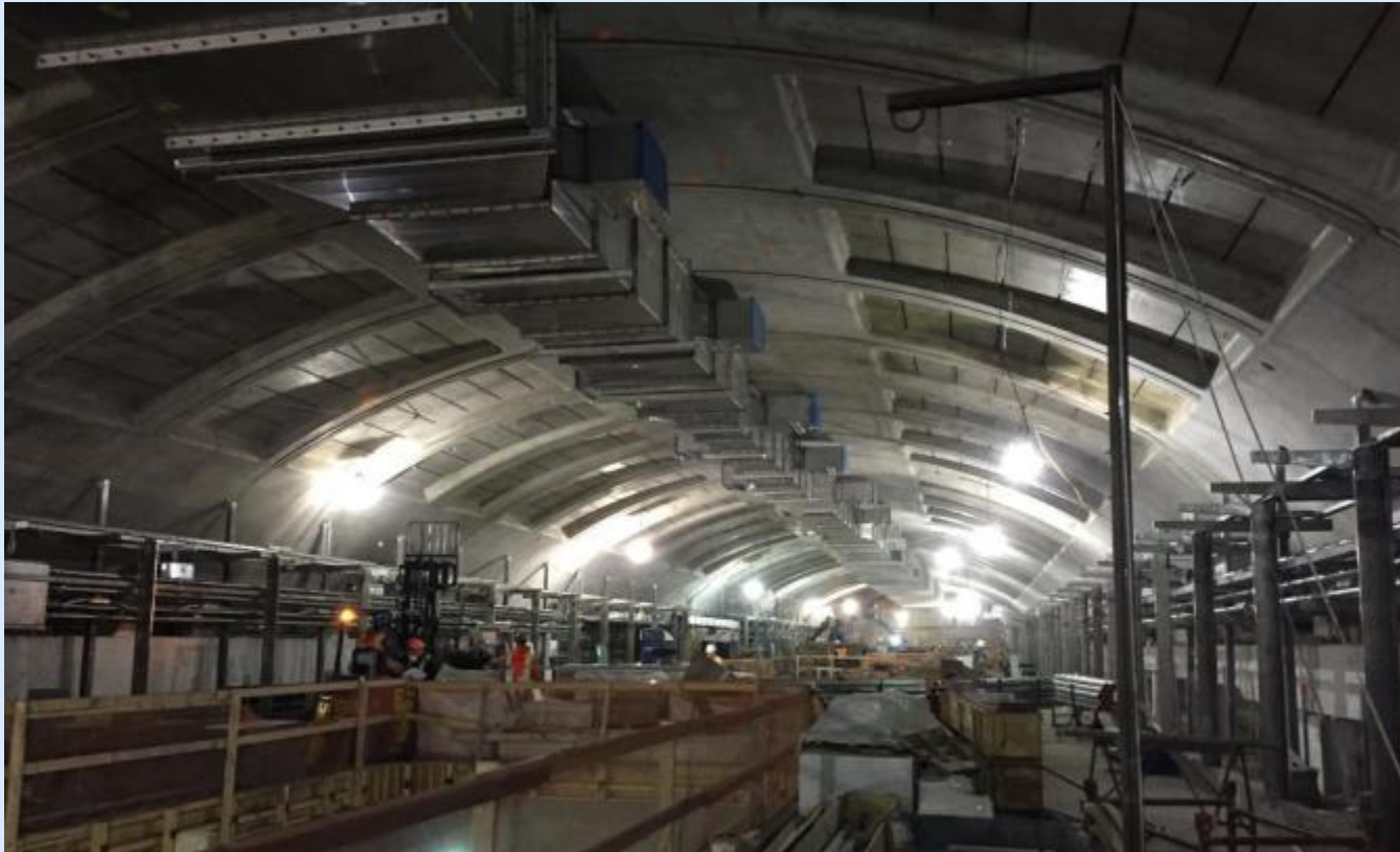
Main Cavern – Mezzanine level wall support framing installation
