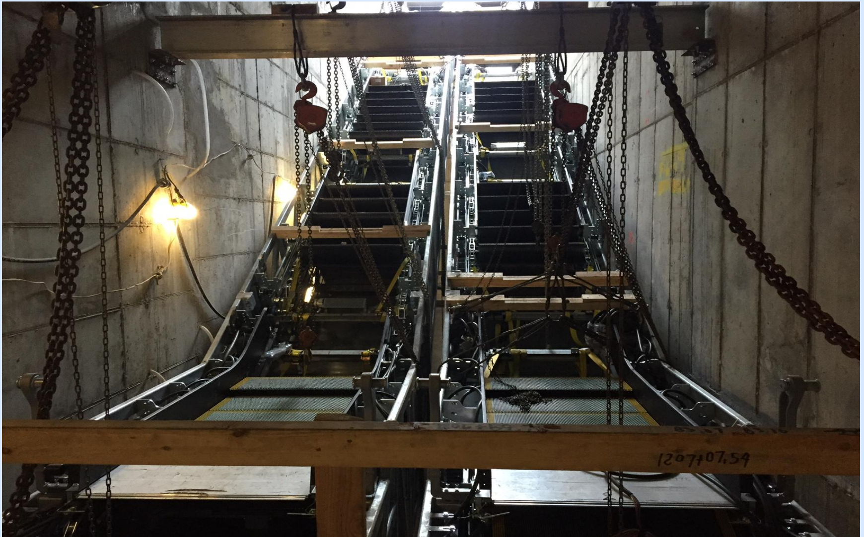
Escalator installation at entrance 2 (86 th Street between Second and First Avenues)
