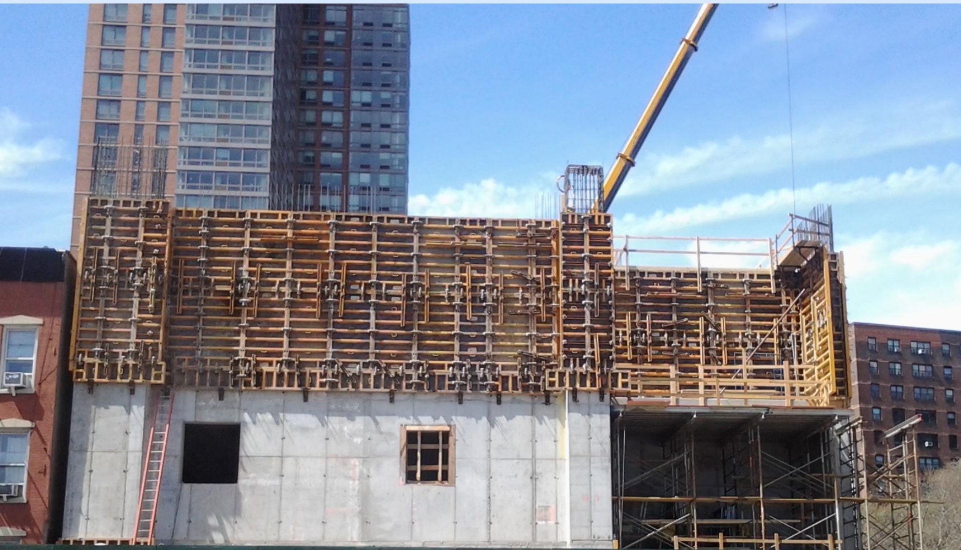
Formwork for Ancillary 2 walls Southwest corner 97th Street
