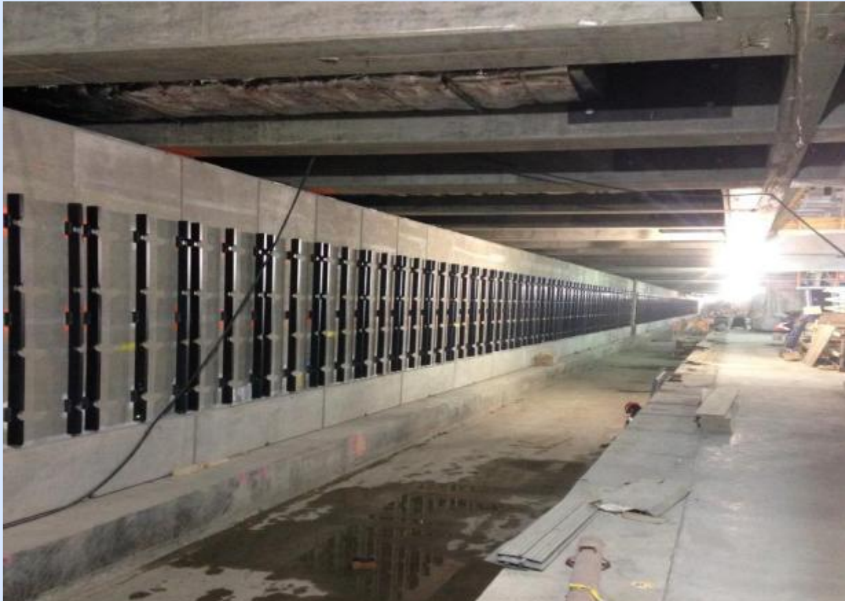
Main Cavern (platform level) – Installation of track wall supports
