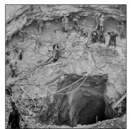
In 1938, a firm from Massachusetts called B. Perini & Sons, Inc., won the \$2.8 million contract to build the temporary cofferdam (a watertight embankment) and a diversion tunnel, which would control the flow of Rondout Creek during the lengthy construction of the Merriman Dam. The method used for stream control on the Rondout Creek differed from previous strategies that were used on New York City dams. The stream control works for reservoirs such as Ashokan and Schoharie had
