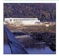
The Holtwood Hydro Power Plant on the Susquehanna River near Lancaster, Pennsylvania is undergoing a \$434 million expansion by adding 125 megawatts of generating capacity to more than double output of the existing 108 megawatts. When completed in 2013, the plant's extra capacity would provide enough renewable electricity to supply 100,000 typical homes. The Holtwood plant has been generating clean, renewable electricity using the flow
