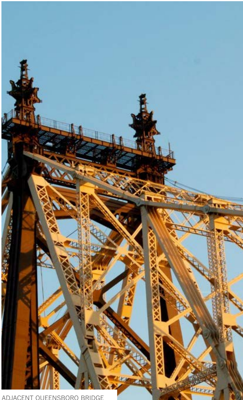
ADJACENT QUEENSBORO BRIDGE
