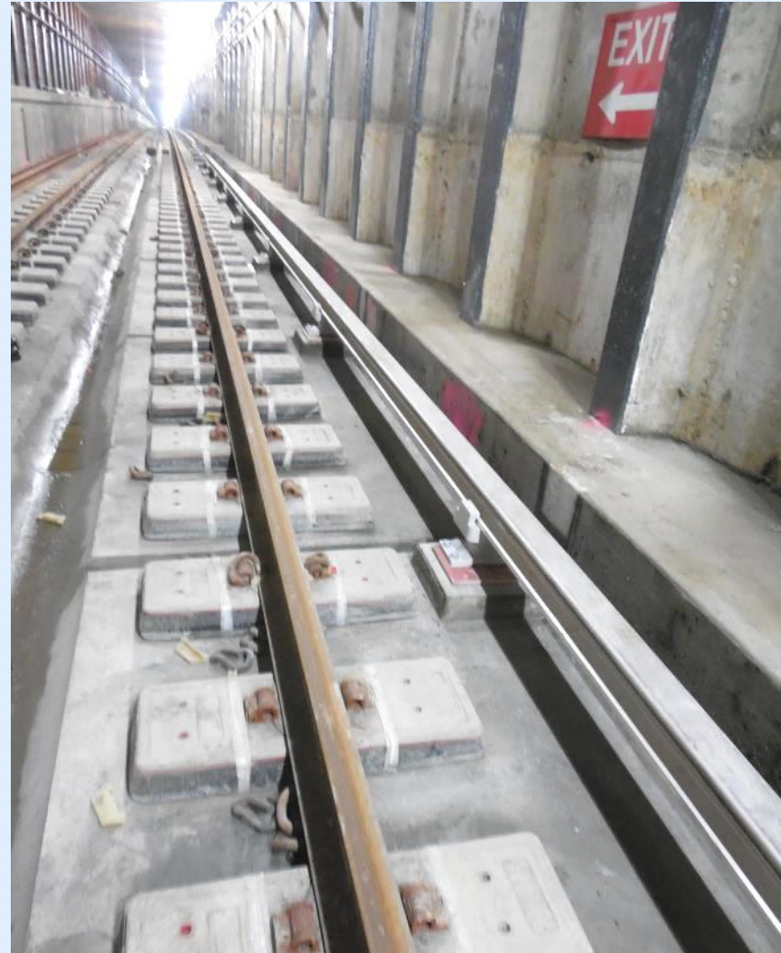
LVT Track installed with Aluminum 3 rd rail
