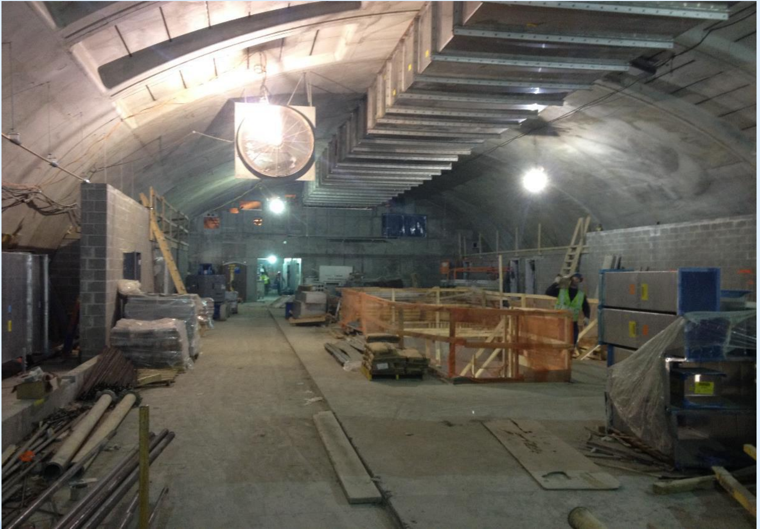
Main Cavern – Mezzanine level masonry wall installation
