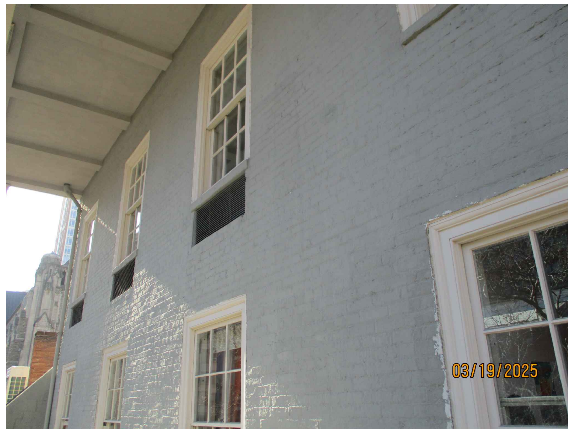
3 EXISTING 4th FLOOR THROUGH-WALL PENETRATIONS
