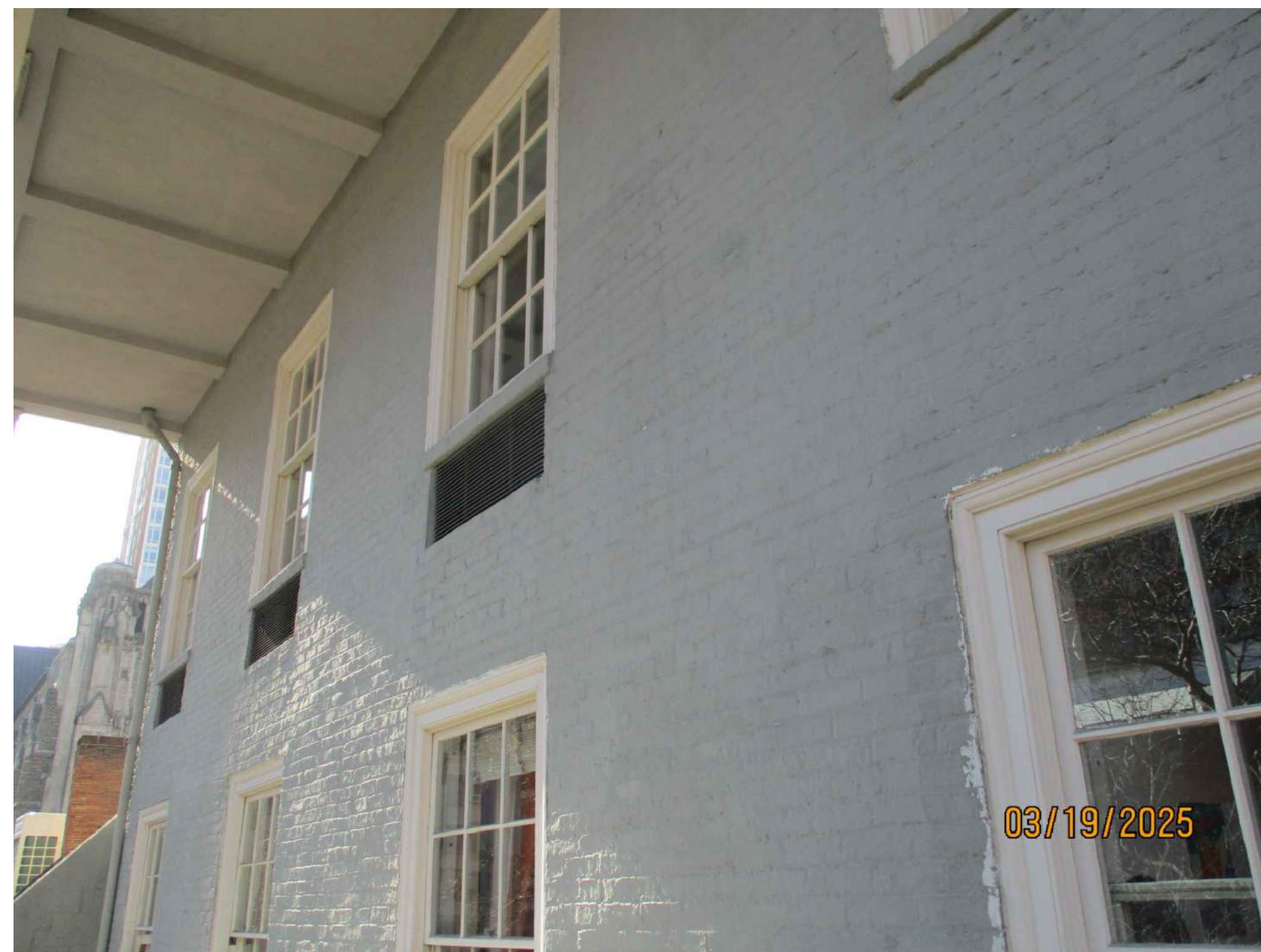
3 EXISTING 4th FLOOR THROUGH-WALL PENETRATIONS
