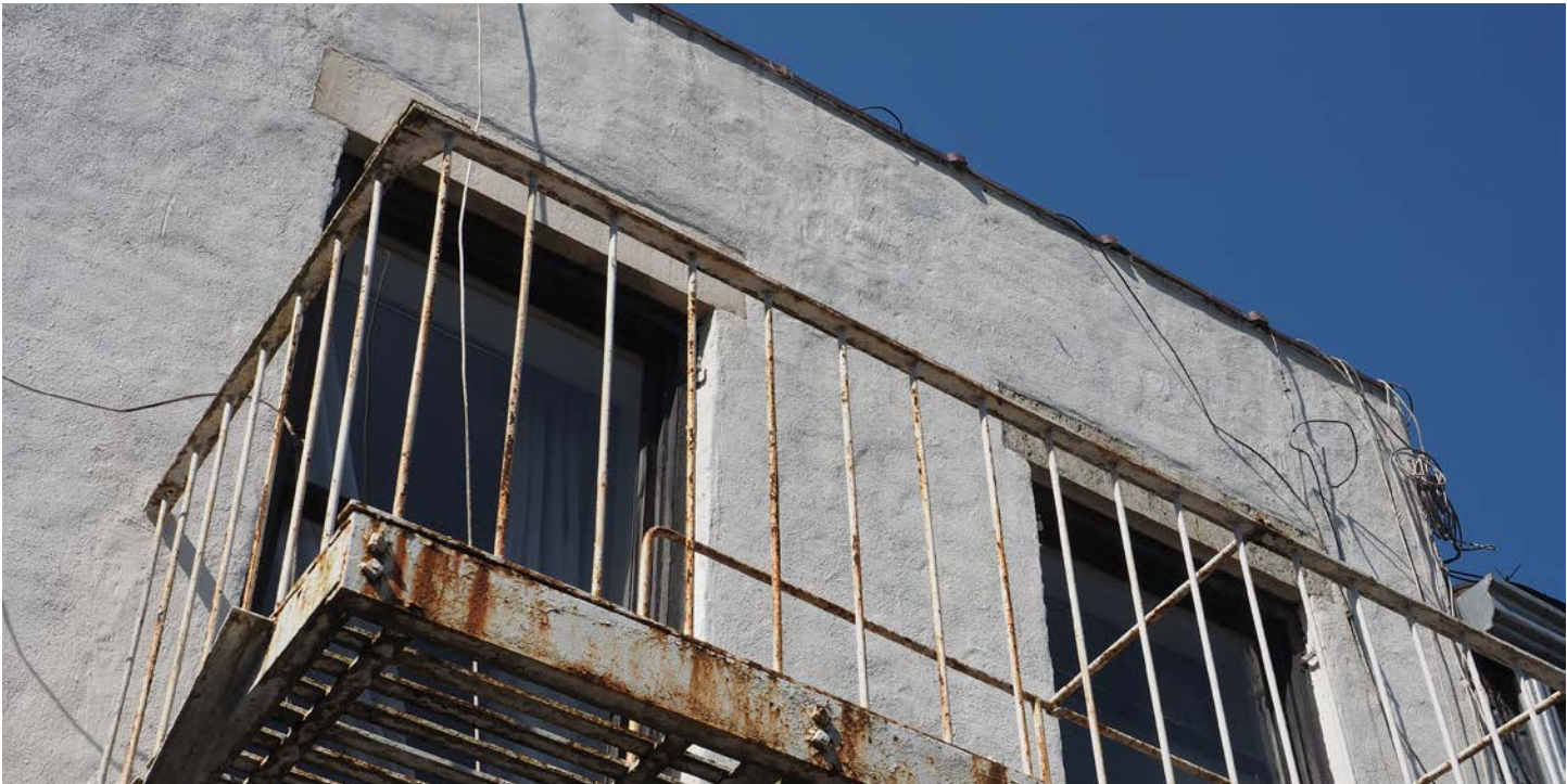
Existing rear fifth-story window openings, fire escape, and parged brickwork.
