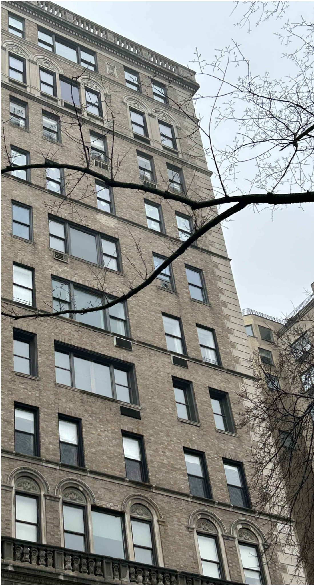
EXISTING WINDOWS PHOTO VIEW LOOKING SE OF FIFTH AVENUE FACADE, FLOORS 5-13
