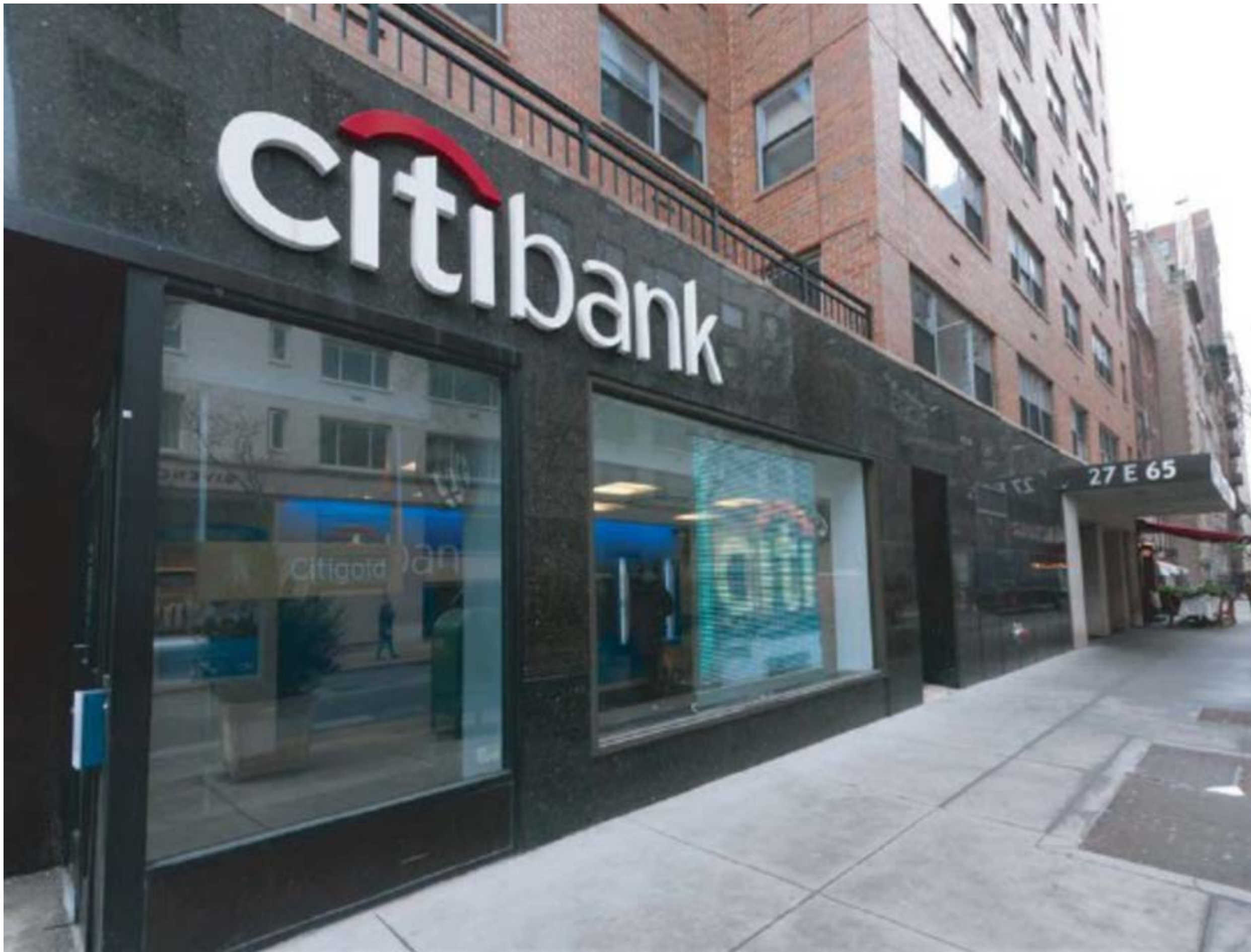
753 MADISON AVE FACADE @ 2017
