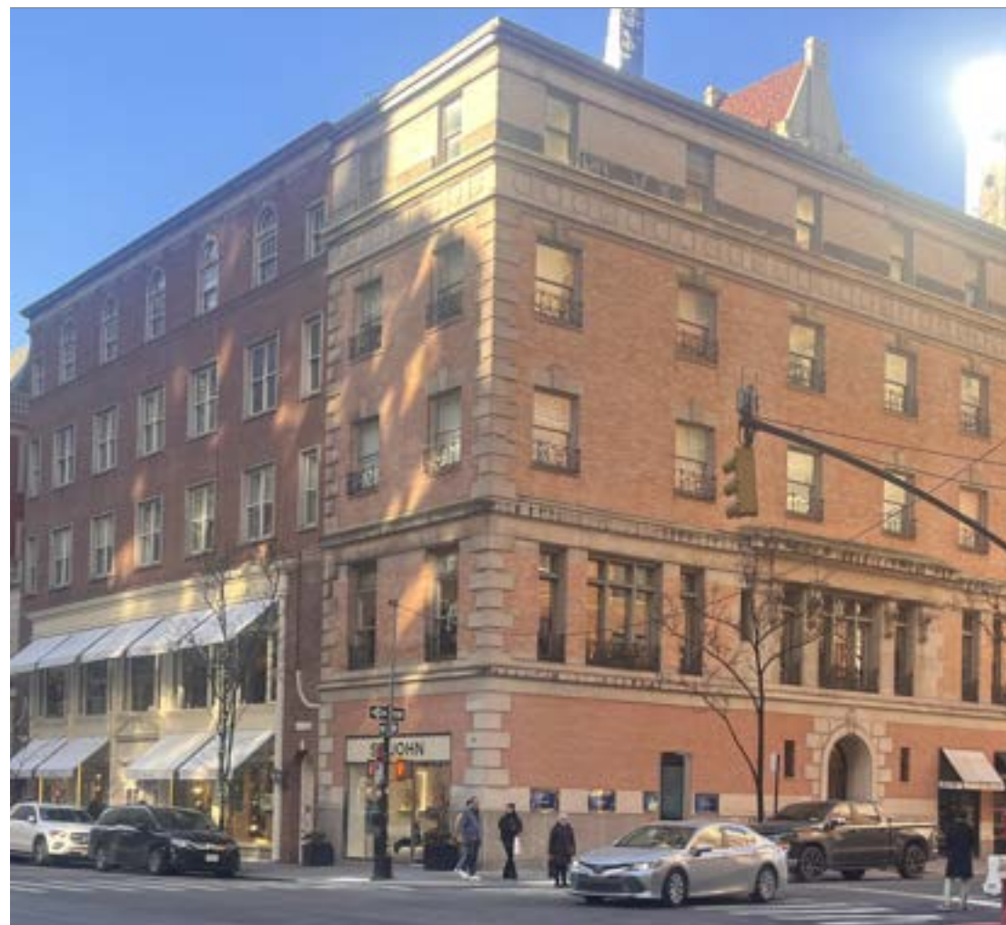
2. ADJACENT BUILDING - CORNER ACROSS SOUTH WEST
