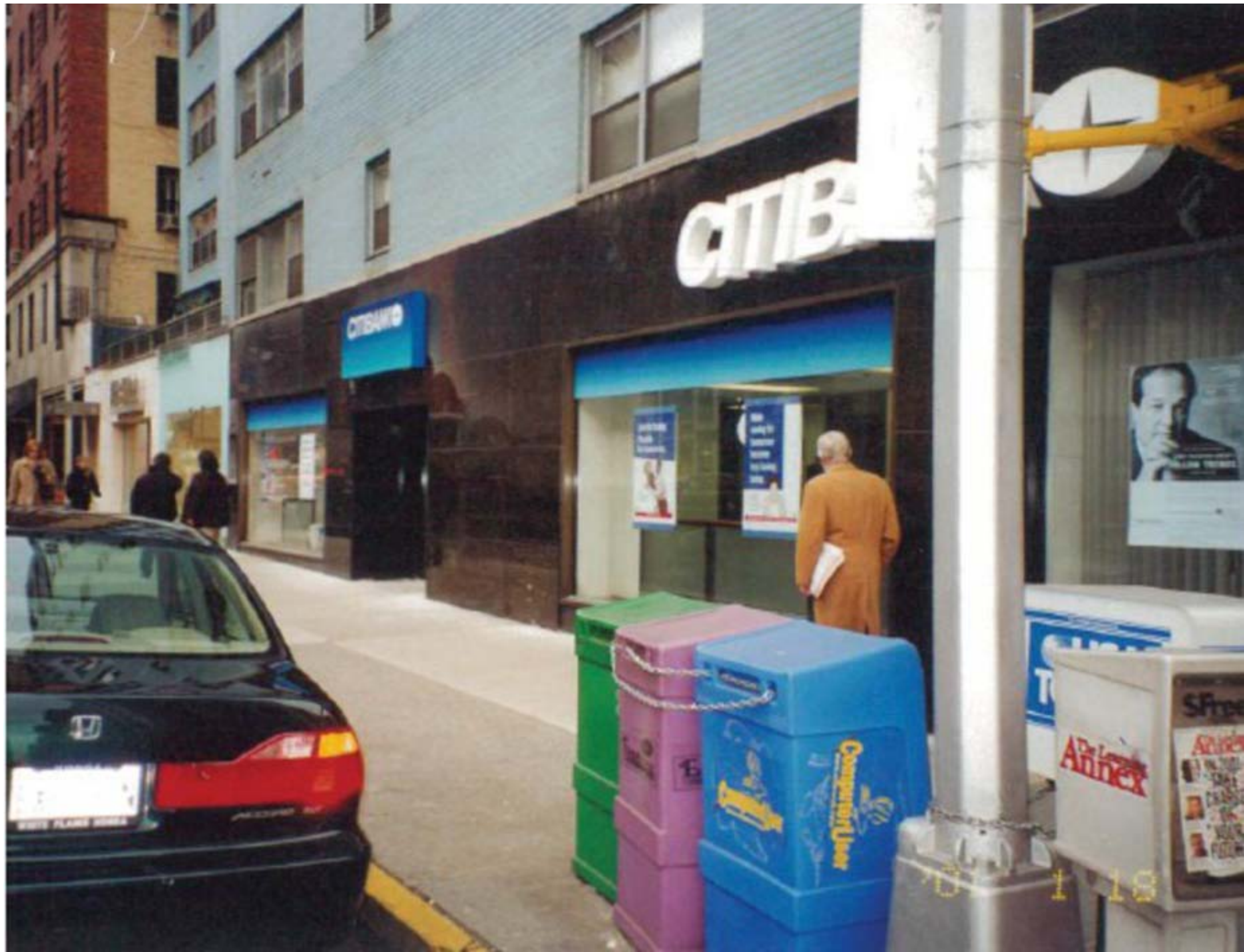
755 & 753 MADISON AVE FACADE @ 2001
