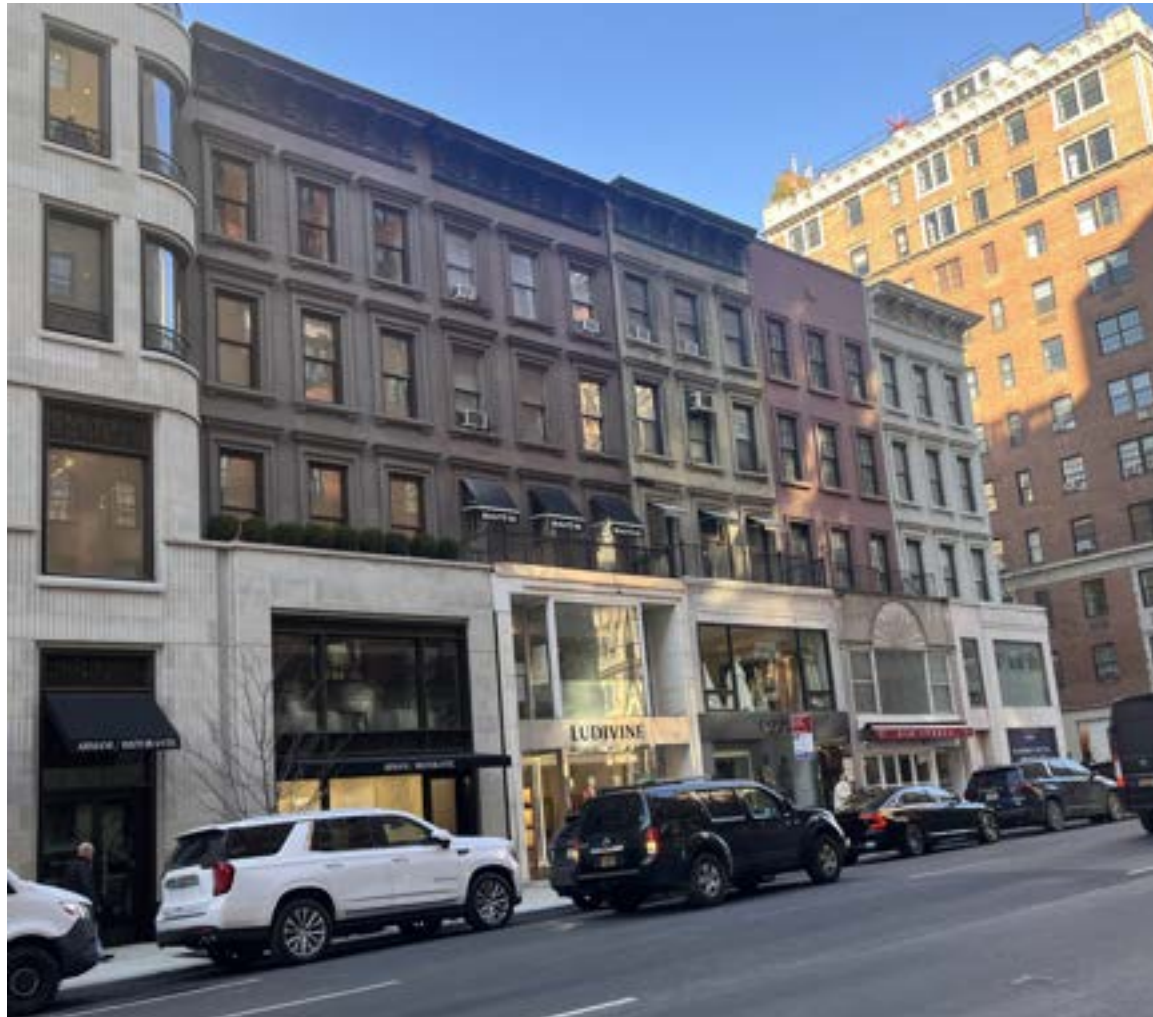
5. ADJACENT BUILDING - ACROSS NORTH WEST
