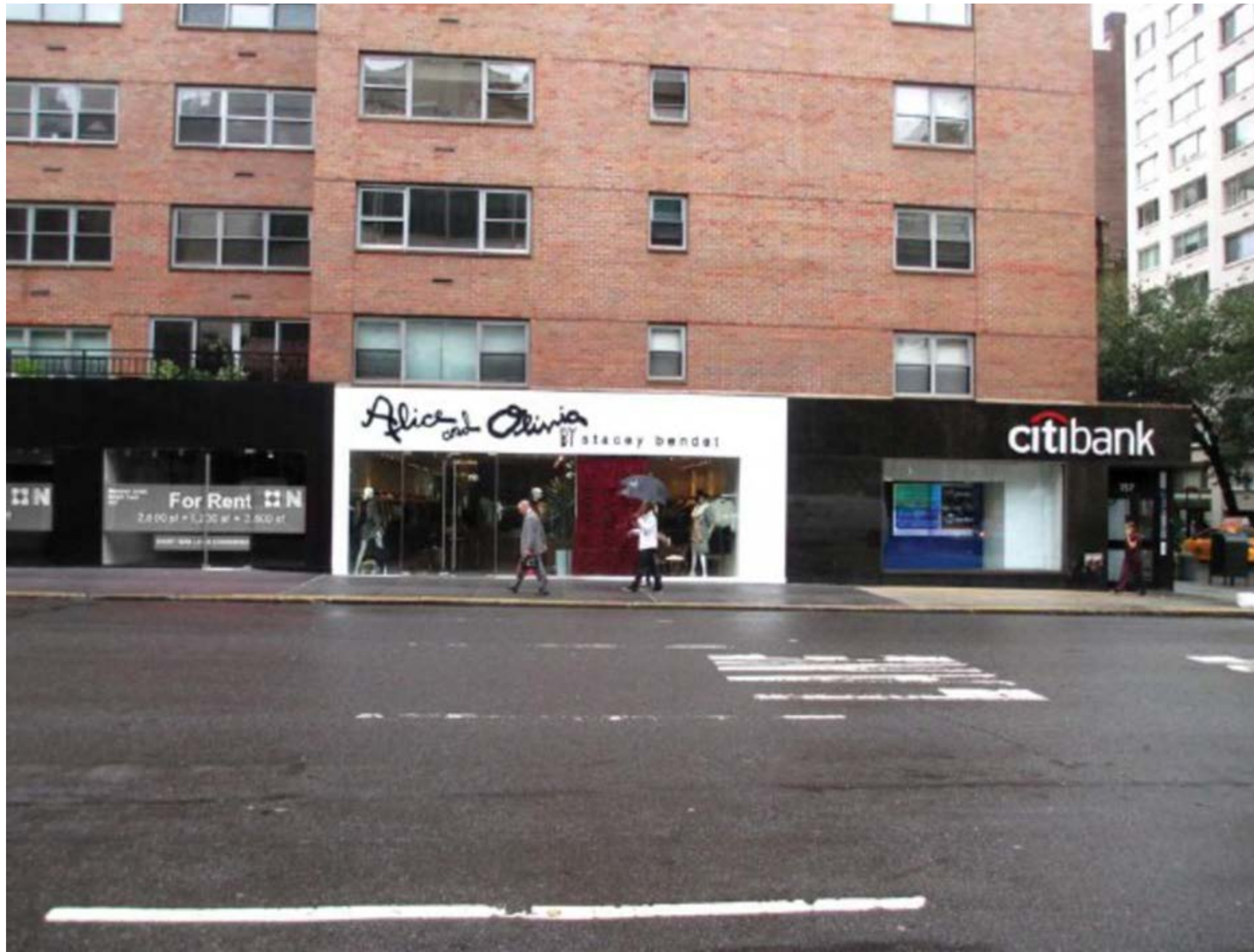
755 & 753 MADISON AVE FACADE @ 2015
