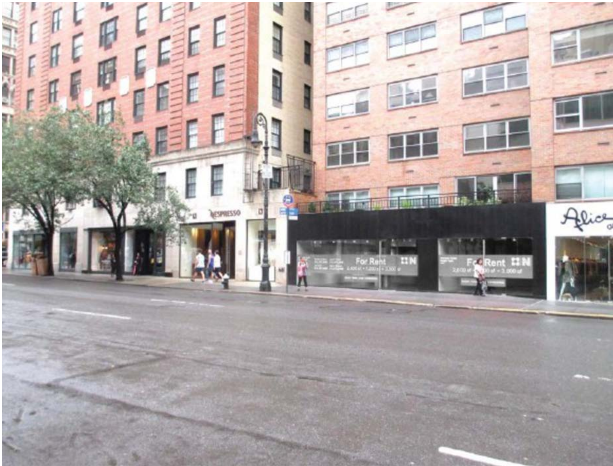
755 MADISON AVE FACADE @ 2015
