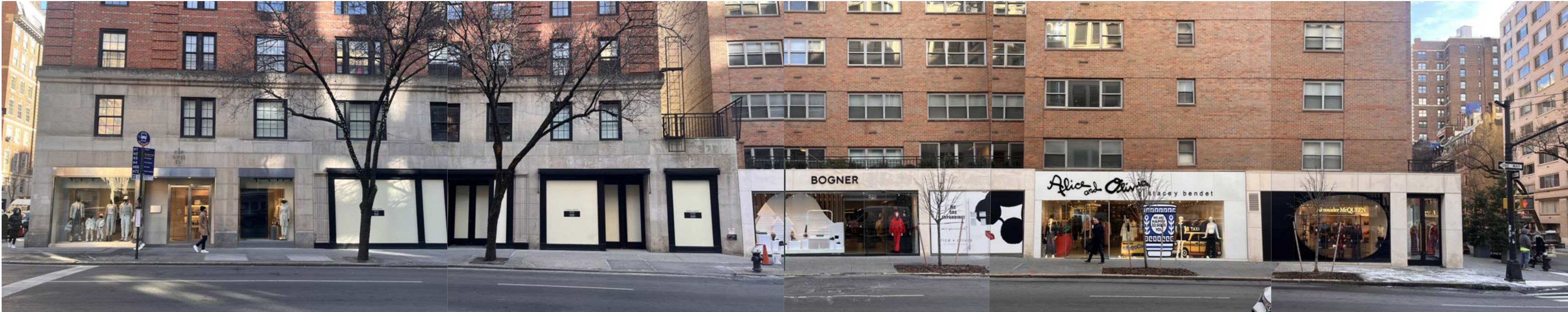
1. ADJACENT BUILDINGS - NORTH & SOUTH
