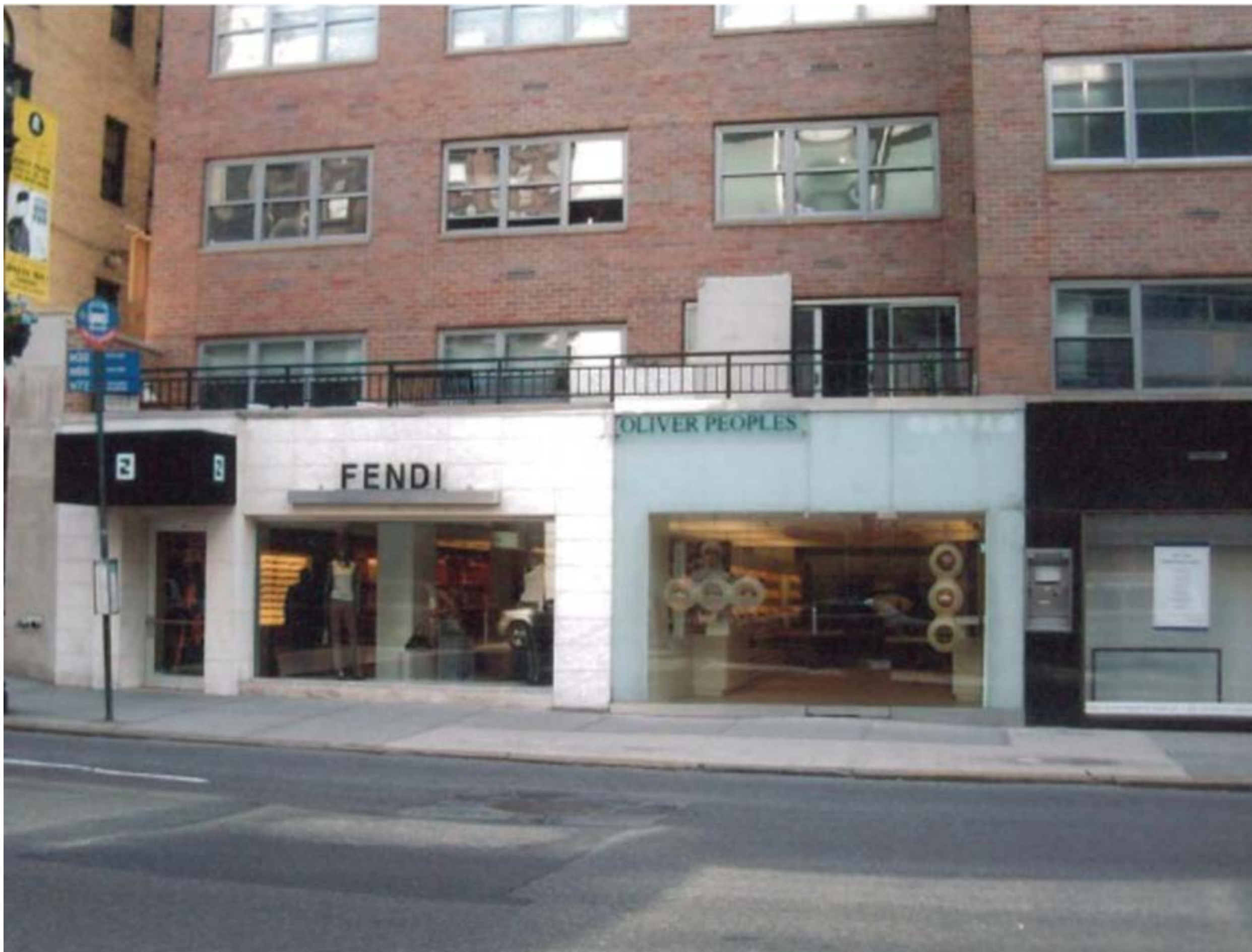
755 MADISON AVE FACADE @ 2005
