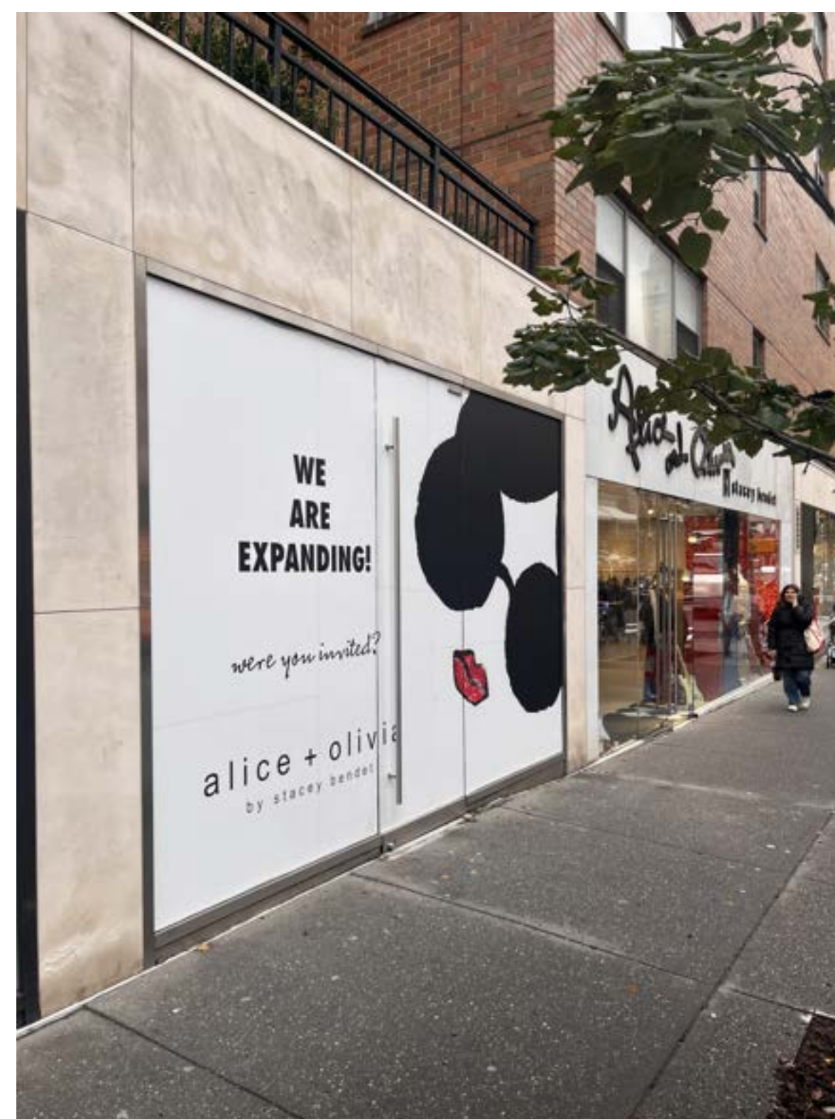
3 EXISTING A+O GROUND FLOOR STOREFRONT PHOTO NTS
