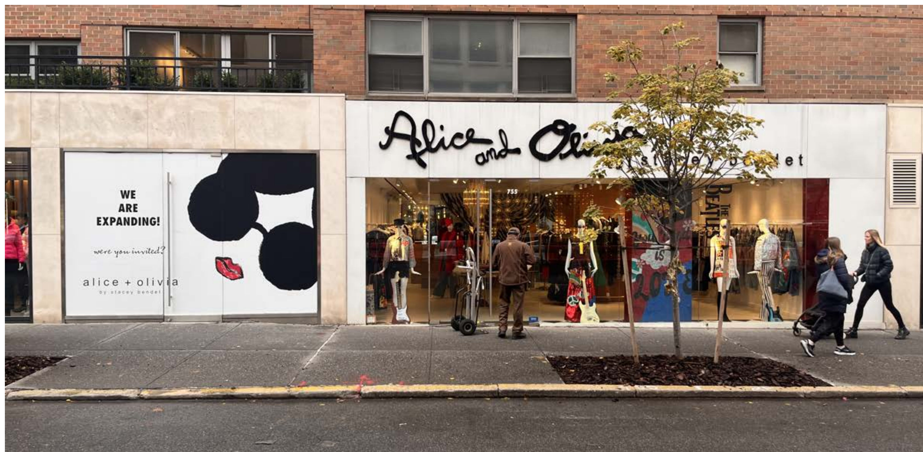
4 EXISTING A+O GROUND FLOOR STOREFRONT PHOTO NTS
