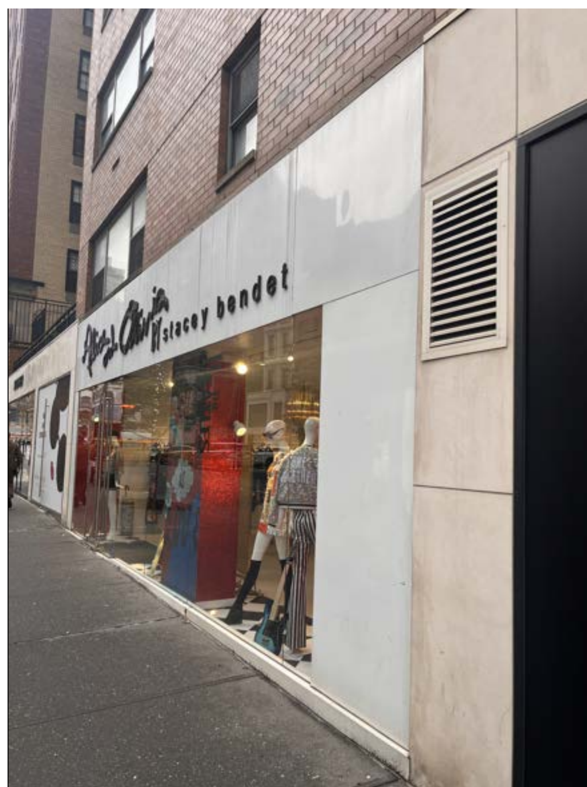
5 EXISTING A+O GROUND FLOOR STOREFRONT PHOTO NTS
