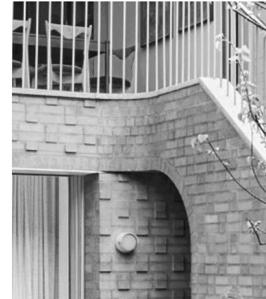
Top to Bottom: Curved brick walls using standard bricks, Double Stoop House, Park Slope, Brooklyn.
