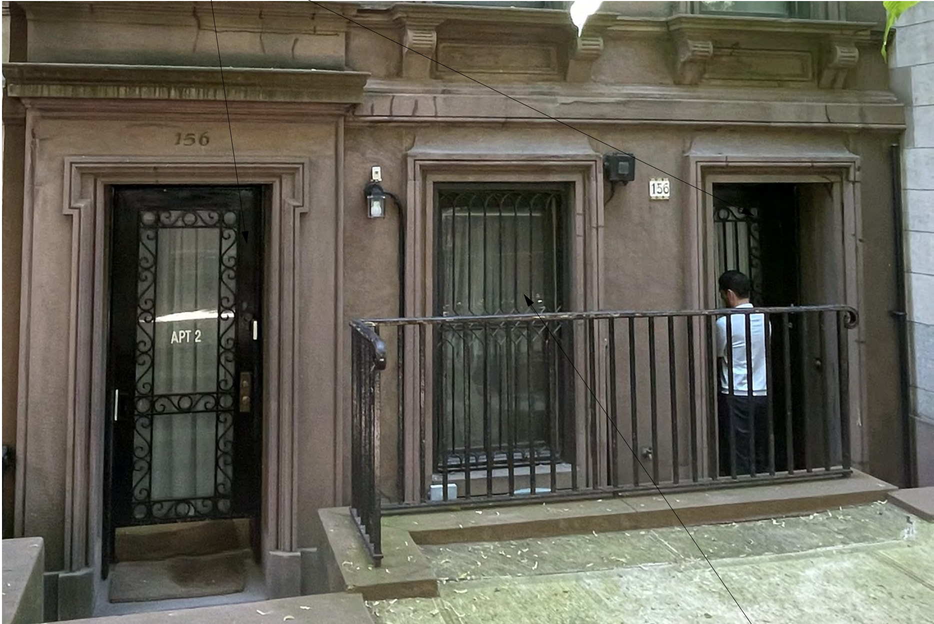
EXIST. BASEMENT FL. WINDOW W/ STONE MOLDINGS & GRILLES
