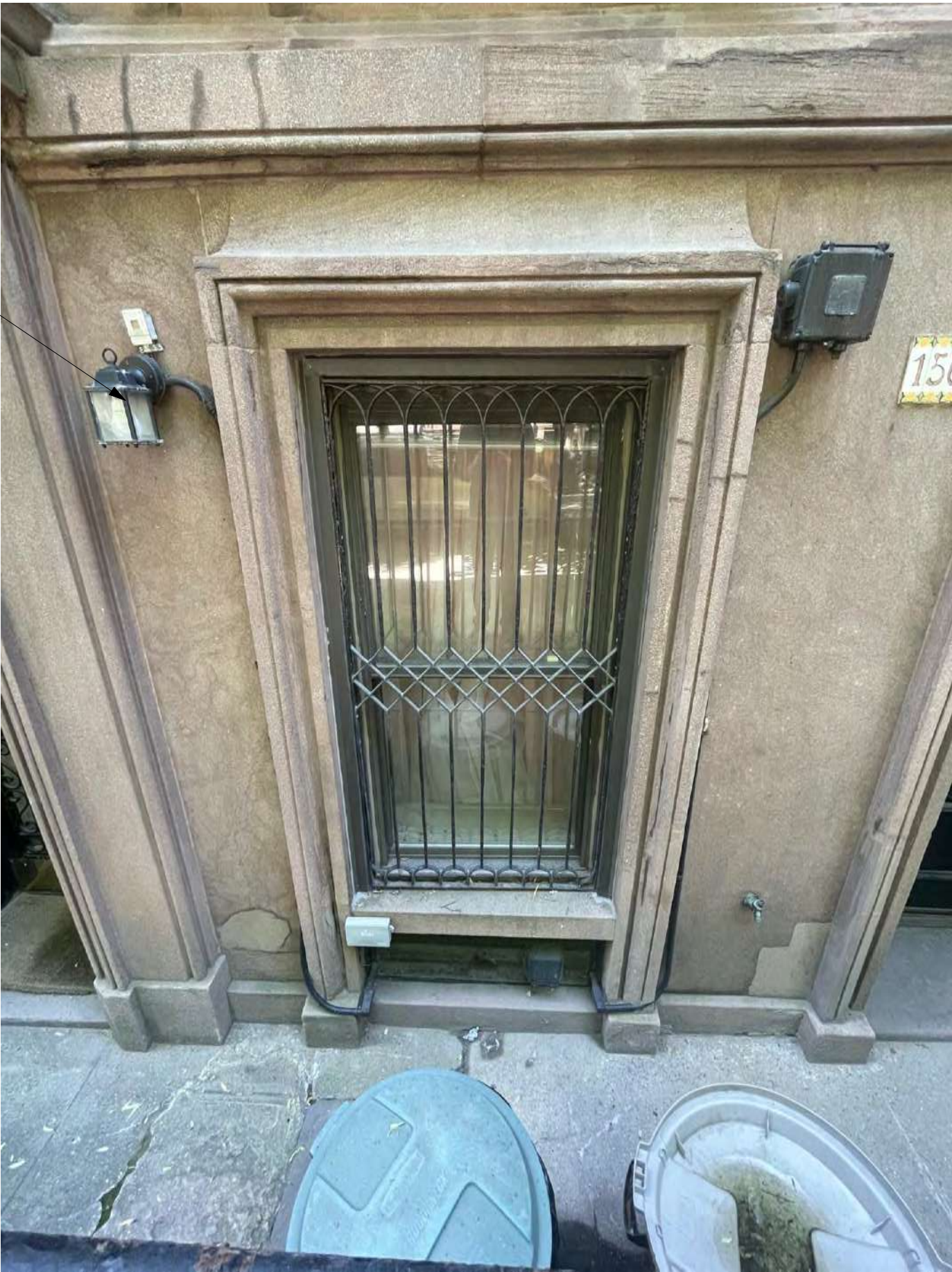
THE EXISTING SECONDARY ENTRANCE DOOR WILL REMAIN AND BE REPAIRED BUT WILL FUNCTION AS A WINDOW RATHER THAN AS A DOOR.
