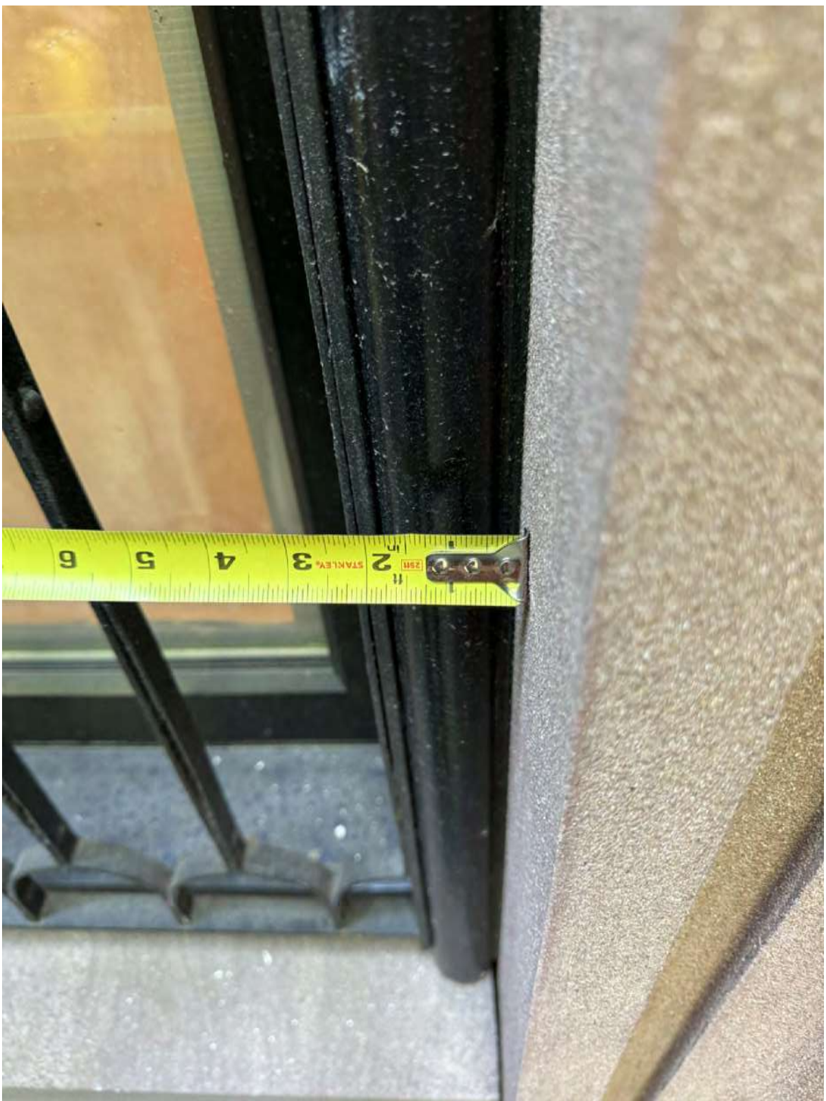
PICTURES TAKEN AT 152 EAST 71ST STREET WITH SIMILAR NEW BRICKMOLD AS PROPOSED
