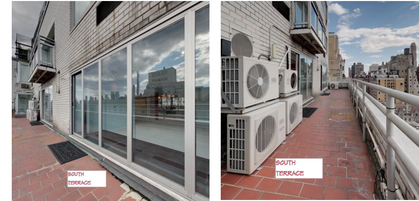
EXISTING PHOTOS OF SOUTH TERRACE
