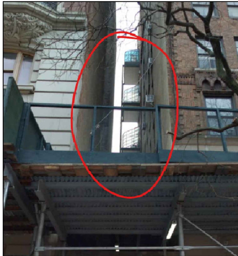
330 WEST END AVENUE (2021) - THE REPLACEMENT OF VISIBLE GREENHOUSES WAS APPROVED, SEEN FROM EAST 76TH STREET.
